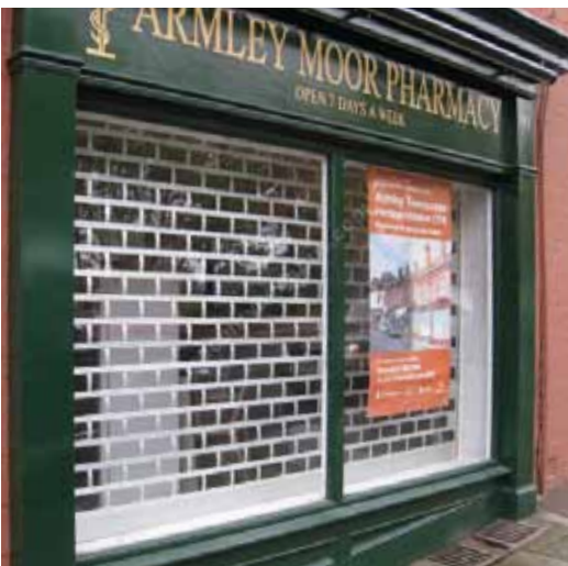
Image of good grill shutter installations
